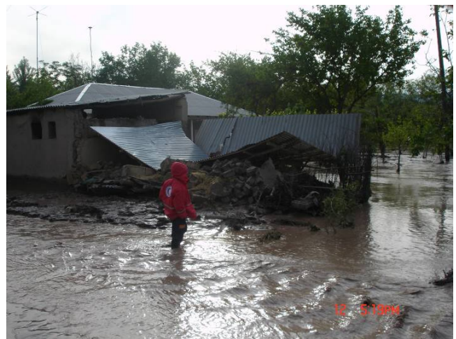
Damaged houses in Vose district. Photo: Shavkat Radjabov, Red Crescent Society of Tajikistan
